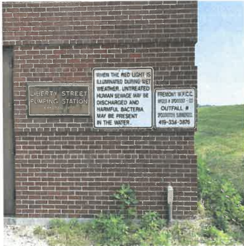
Pumped CSO Location
